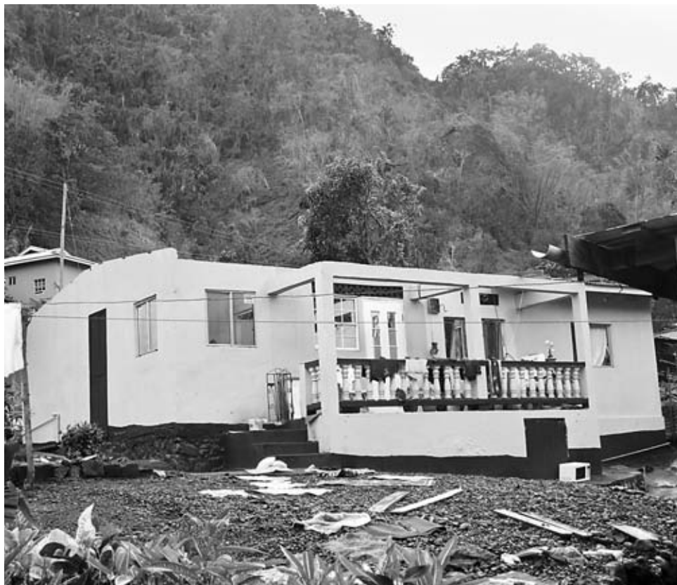
ONE OF THE many houses left roofless in Chateaubelair after the passing of Hurricane Tomas
