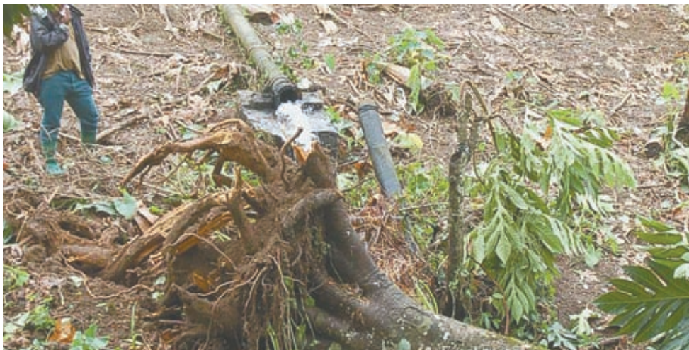
A SECTION of the massive breadfruit tree which fell and severed the CWSA Montreal water main, disrupting service.
