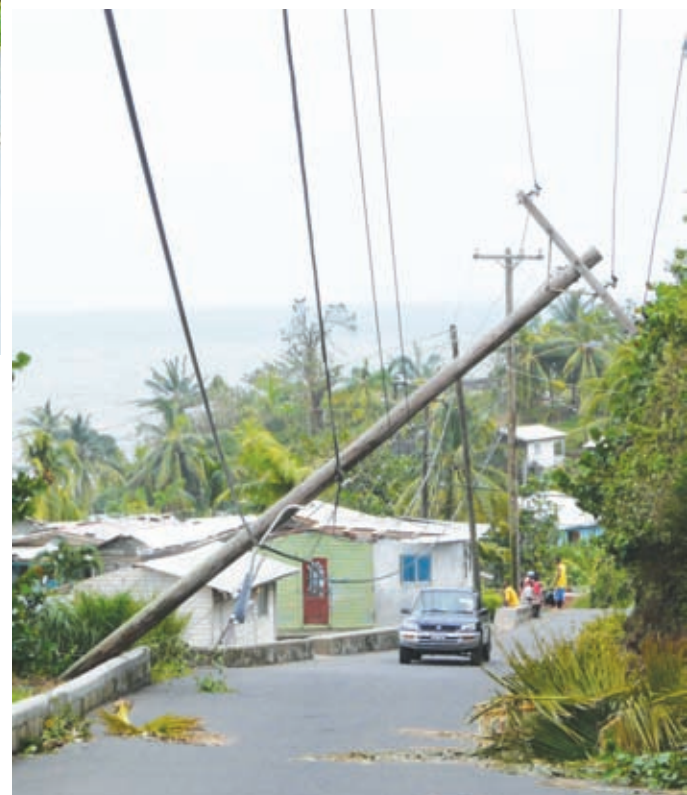
THIS pole is seen here leaning after the passing of Hurricane Tomas.
