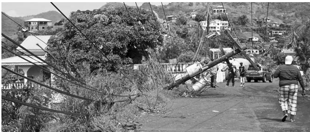
DOWNED ST. VINCENT Electricity Services Ltd. (VINLEC) pole, carrying high tension wires and a transformer, close to where Burgess lives.
